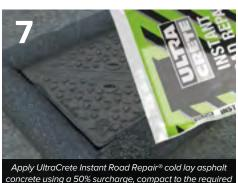
depth (typically 45mm layers, compacted to 30mm)
